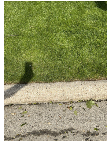
Well maintained curb:
